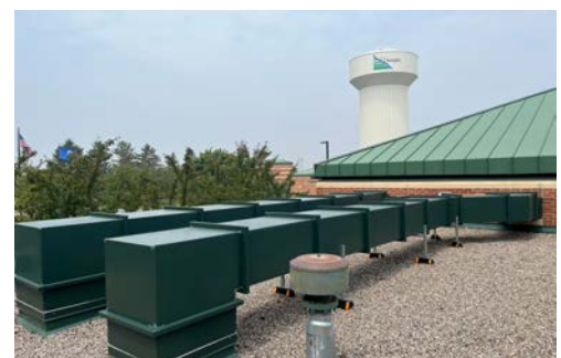
Pro-R Specialty is a pre-insulated duct solution suitable for outdoor and indoor applications.
